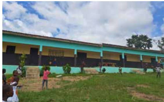
A complete new school in Allakouadiokro
