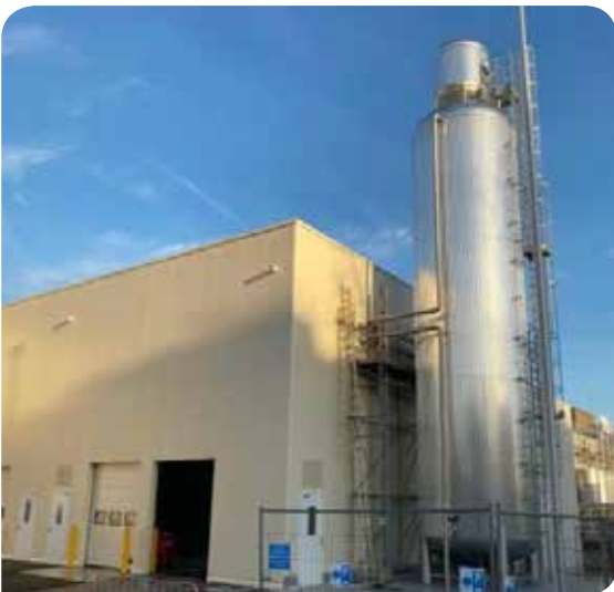
Hot water grid - 85% complete
